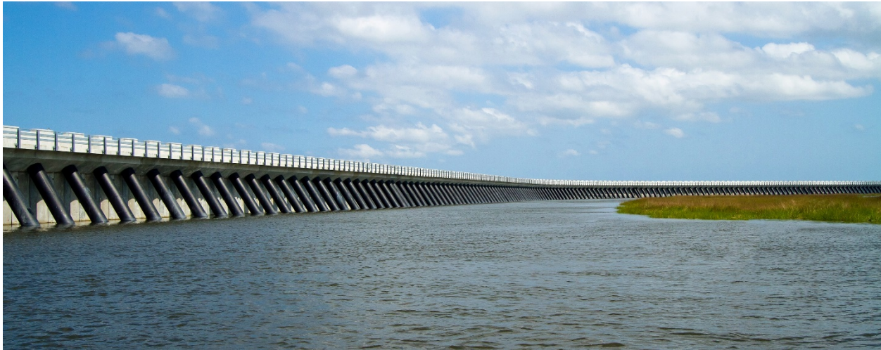
Figure 3-2. The Inner Harbor Navigation Canal Surge Barrier in New Orleans is an example of a combo-wall. It is built to approximately 26 feet (NAVD88).
